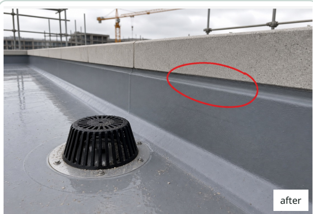
Roof drain membrane edge marked after remedial seal.
