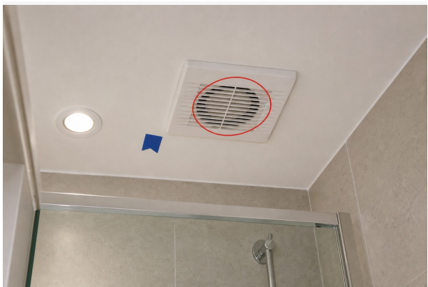
Extractor fan did not operate during the check. Captured 2026-07-10 12:00 - SHA-256 2136a76d2077bad4 (verified)
